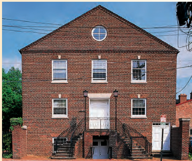
This Scottish Presbyterian Church, built in 1794, still stands in Alexandria, Virginia.
